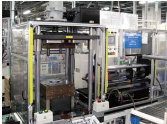
Kangawa Works Factory equipment installation
